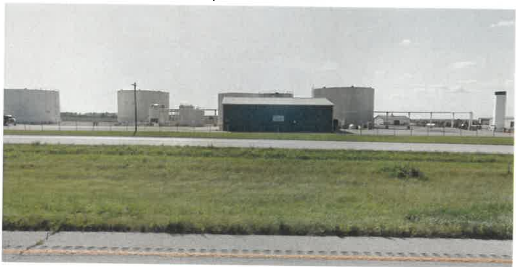
Figure 5: Magellan Pipeline Company Breakout Station
