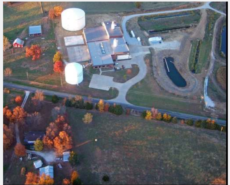
The CCWWC drinking water treatment plant draws water from the North Fork of the Salt River.
