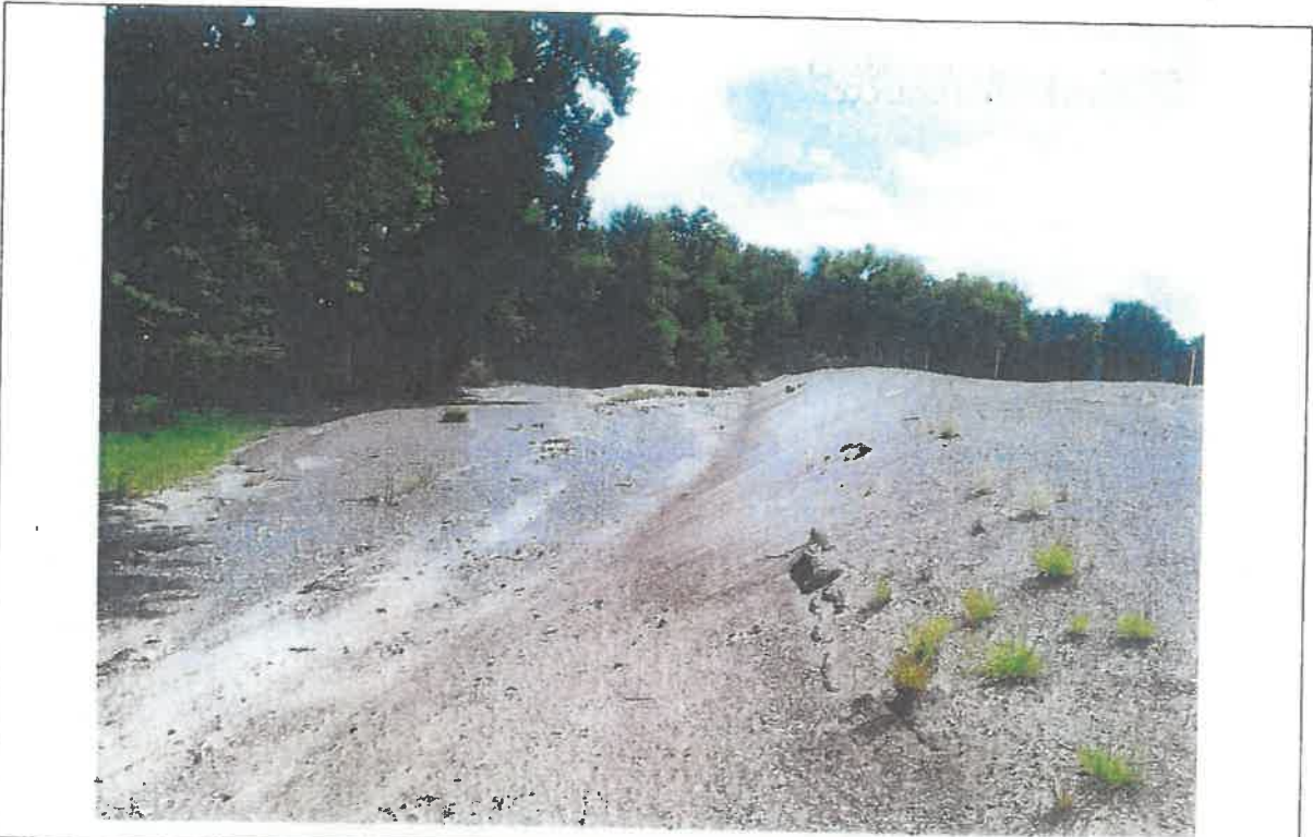
Photo 1: Typical scour damage facing downstream
