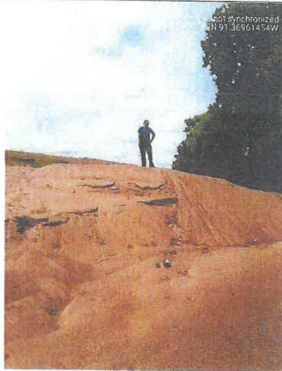
Photo 6. 13 foot tall sand pile deposited at downstream end
