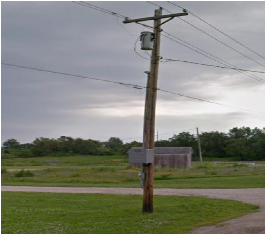
Sparklight Powered Cable node on the north side of La Plata
