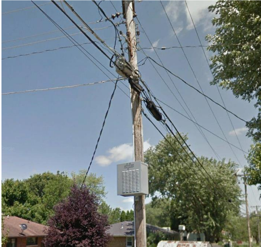
Charter Communications (Monroe City) coaxial cable amp and Fiber over lashed to existing cable strand
