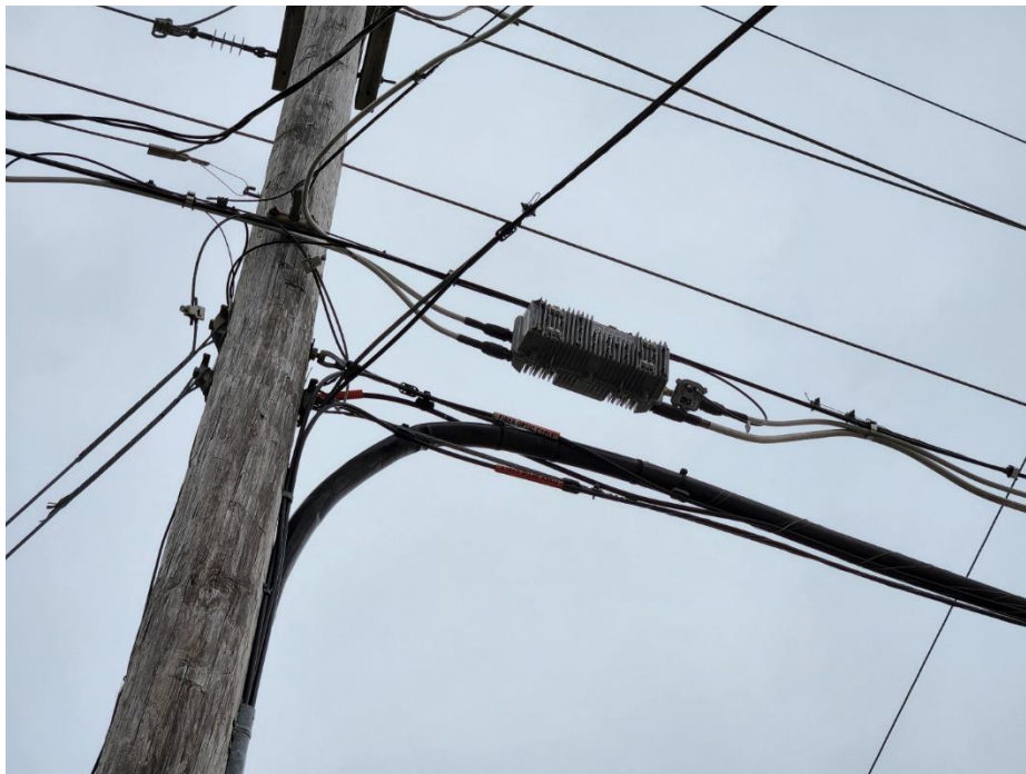
Charter Communications (Monroe City) coaxial cable amp and Fiber over lashed to existing cable strand
