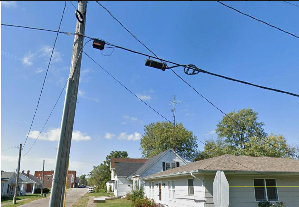
The picture above is of a Yondoo fiber cable and drop installation in Bowling Green.
