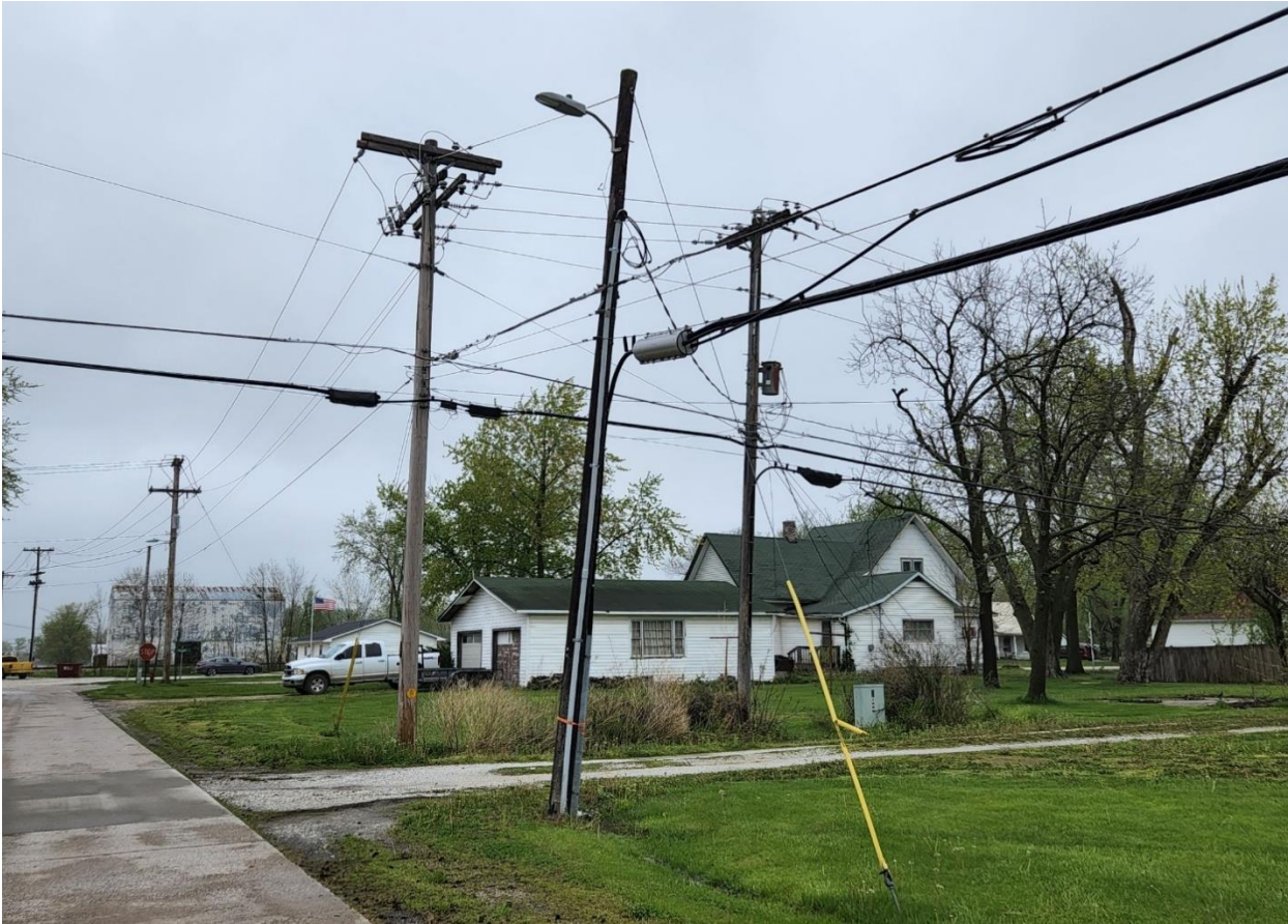
Charter Communications (Shelbina) fiber over lashed to coax cable and existing cable strand
